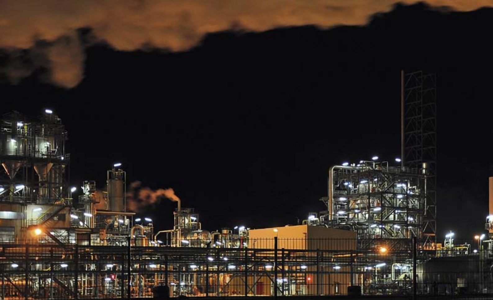
The cracker in Böhlen is the centrepiece of the chemical site.
