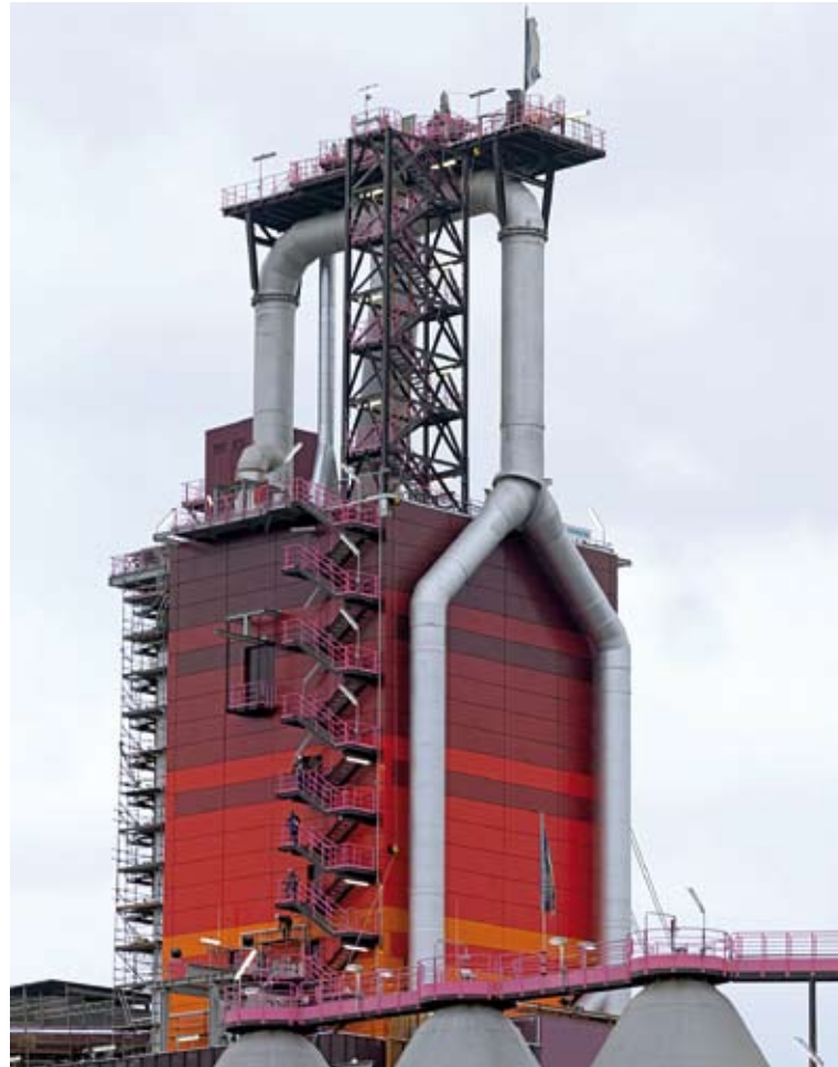
Blast furnace 8 in the Duisburg plant was commissioned in 2007 and produces around 5,600 tonnes of pig iron every day
