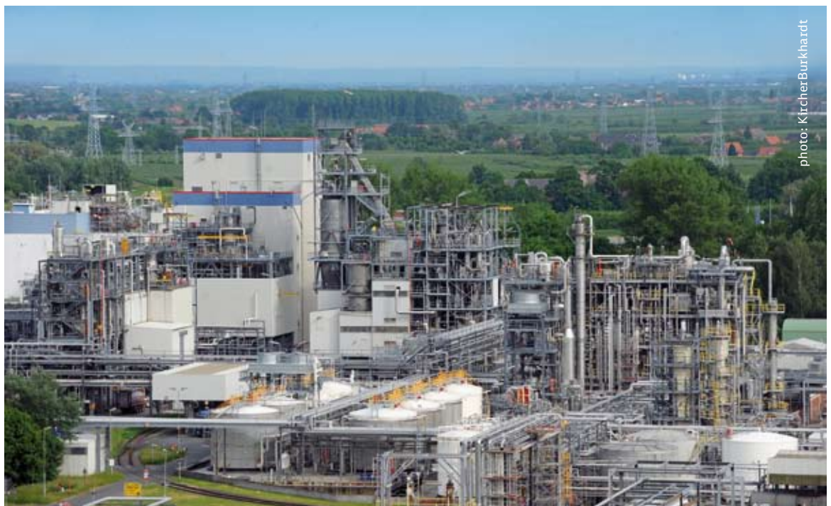
With 16 production plants on a site of 550 hectares, the Dow facility in Stade is the second-largest location of the chemicals company in Germany
